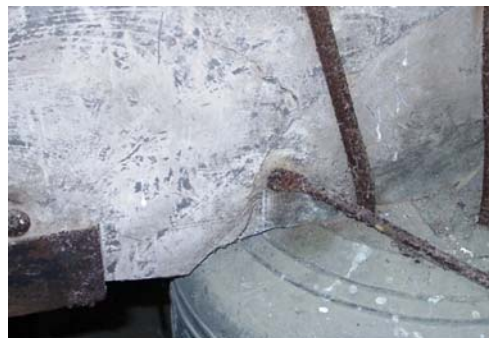
The cracked headstock of the 3 rd bell
